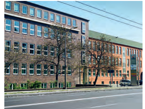
↑ Ardel's company premises in Eberswalde
