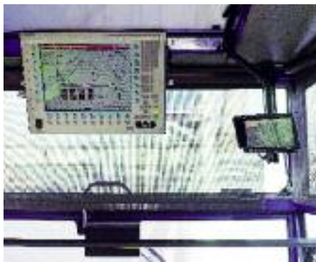
↑ Visualization of crane data via the crane-management system
